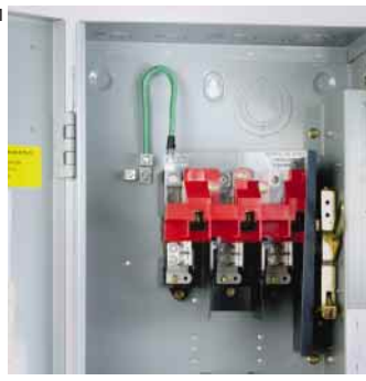
1. Double Throw Switching Neutral Safety Switch (upper switch base assembly is shown)
